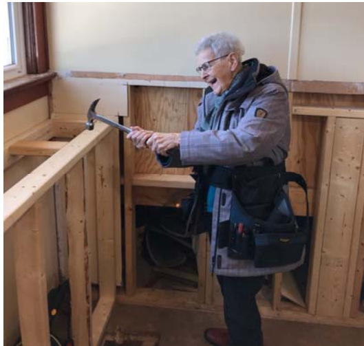
Sister Phyllis helping put the new elevator in.
